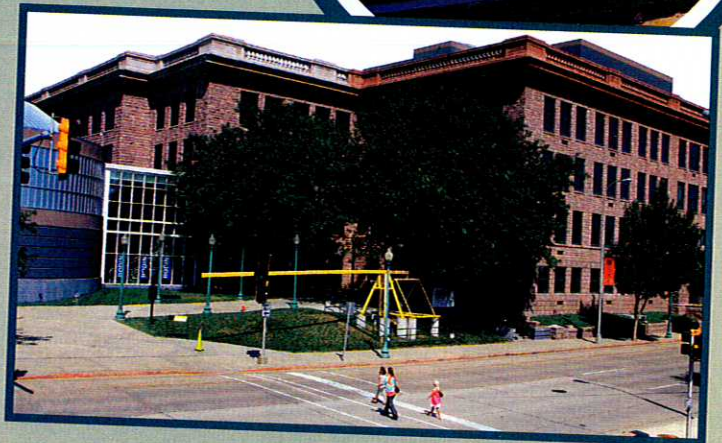
Renovated building: Washington Pavilion
